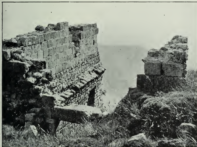
FIG. 238.—Kizil Hissar, two-storeyed building.
